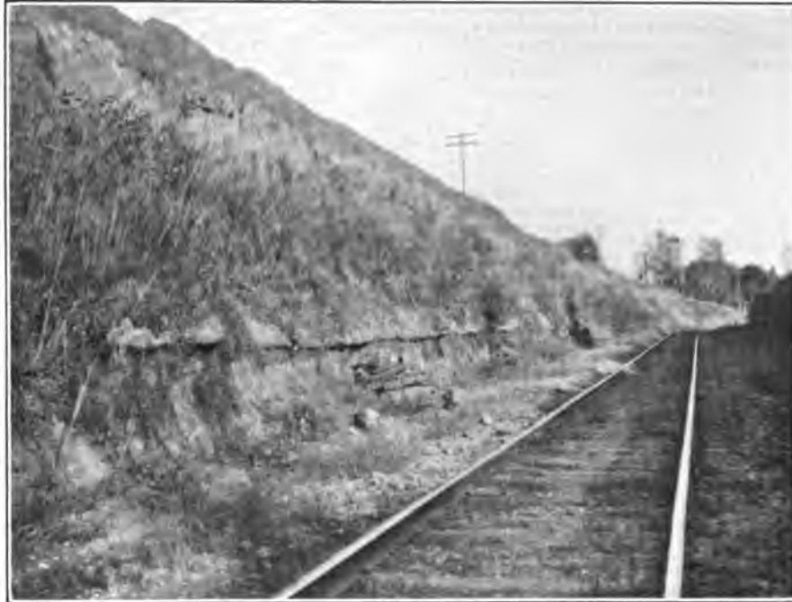
A. CRETACEOUS-EOCENE CONTACT IN CUT OF ST. LOUIS & SAN FRANCISCO RAILROAD 1 MILE EAST OF NEW ALBANY, MISS.
